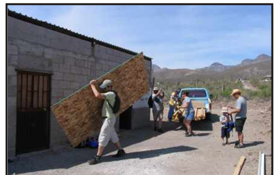
The builders team construct a Medical Clinic.
